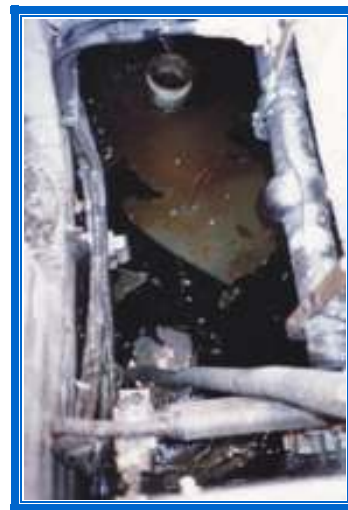
The Solidified oil is lifted off the water surface in a rubber sheet
