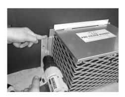
Place Pre-Filter basket against wall around Petro-Pipe. Put the 'Z' brackets against the Pre-Filter flange and drill holes.
