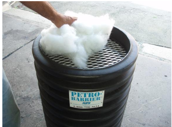
Inspect the cavity and clean out any dirt and debris. Re-pack with new floss and GSE fabric. Replace metal grate and retaining ring .
