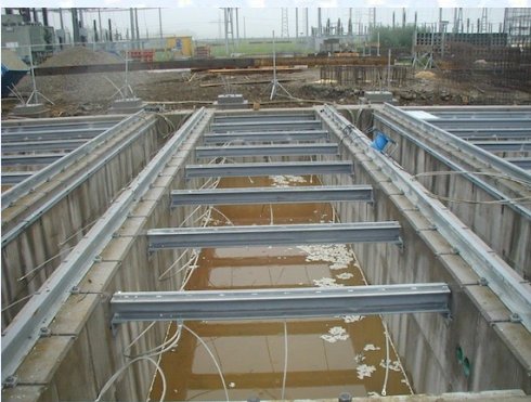
Support system designed for Concrete Containment Pit and StoneQuench™ LHD® Grating.
