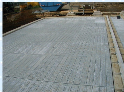
StoneQuench™ LHD® gratings are easily installed on the supports providing a dirt free - Fire Extinguishing System.
